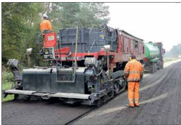
Abb. 11: Kaltrecycler WR 4200 – Kaltrecycling in-situ (Foto: Fa.Kutter GmbH)
